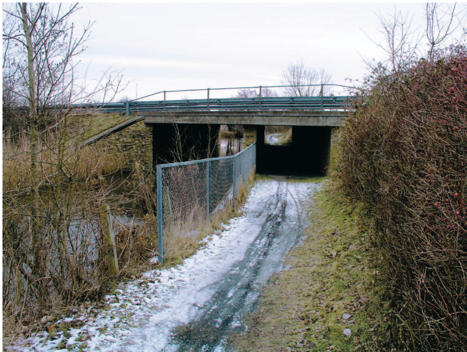
Figure 5. Reinforced concrete slab structure.
